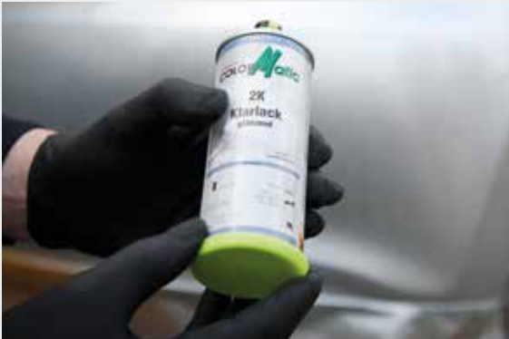
1.Remove protective cap.
